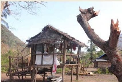
Figure 1 Damaged houses in the Tagbanua communities
